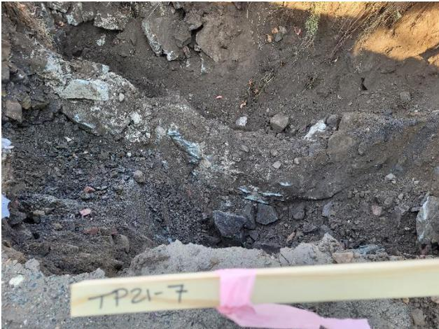
*Photo 18: Image of former concrete foundation element observed in TP21-7, looking south.*
