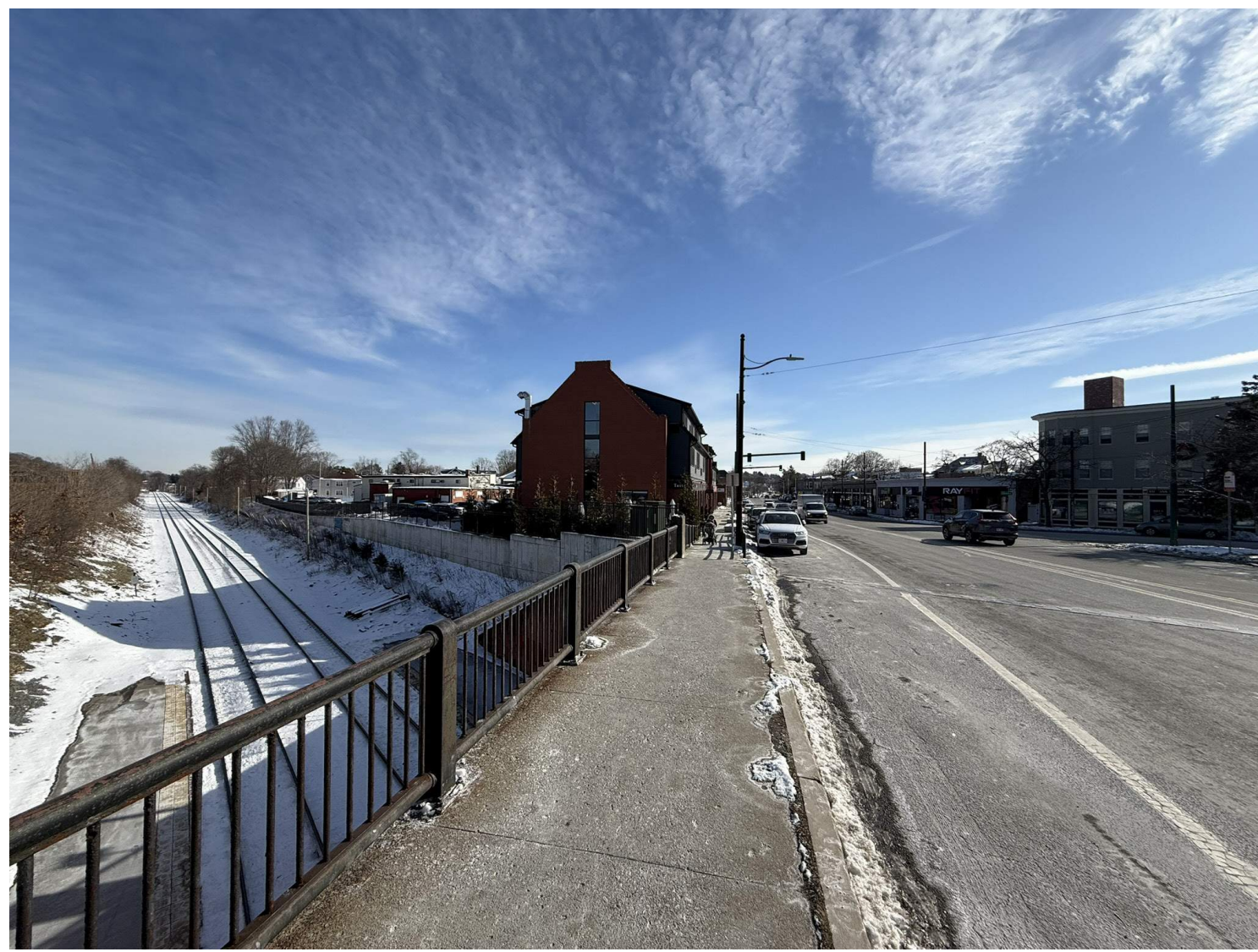
TRAPELO ROAD BRIDGE ABOVE MBTA
